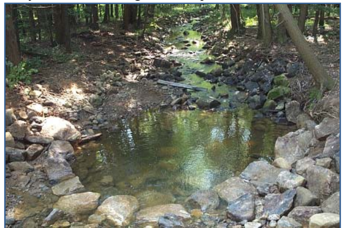
Crossvane weir installed below bridge to create pool habitat for brook trout.
