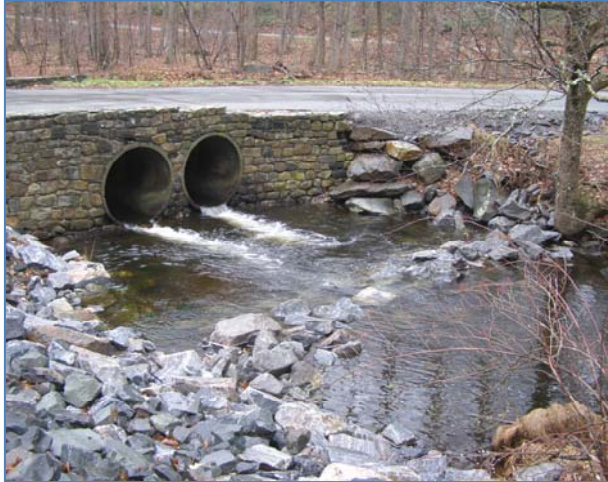
Perched twin culverts on Lake Waramaug (Sucker) Brook. Installation of a vortex rock weir immediately downstream of the Town Hill Road bridge increased water surface elevation, providing upstream fish passage by backflooding the culverts.
