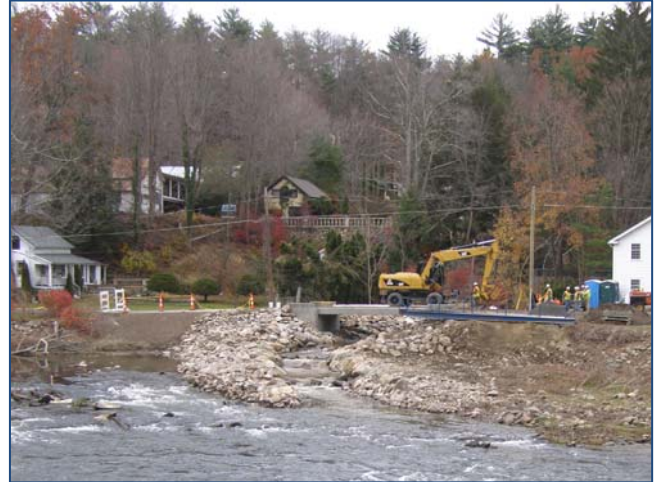
The enhanced channelization at the mouth of Mill Brook is intended to redirect and concentrate cool water inflow to improve the thermal refuge at the confluence with the Housatonic River in Cornwall.
